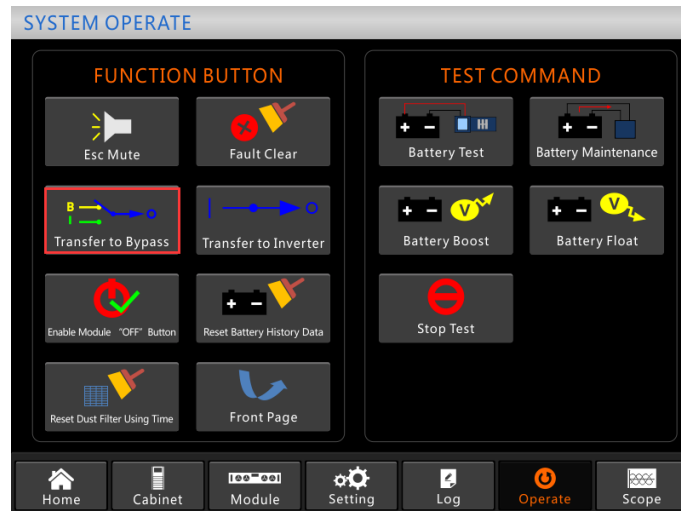
The operation interface for transferring to bypass
